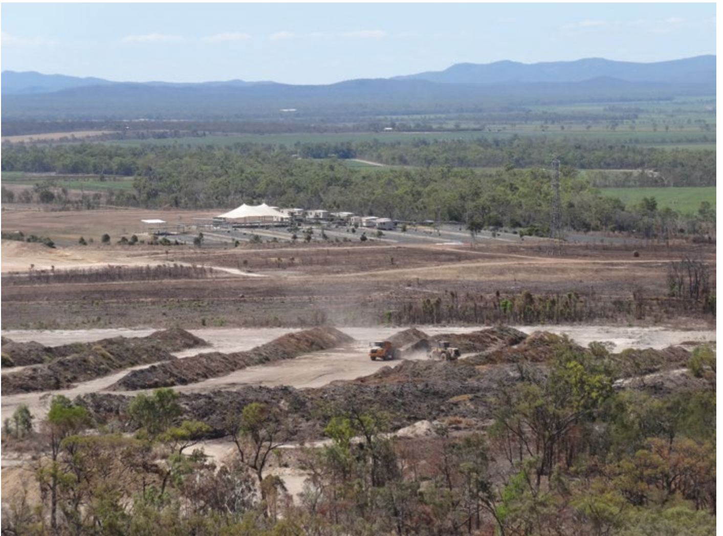
Cover: Lake Macquarie ORRF during construction
