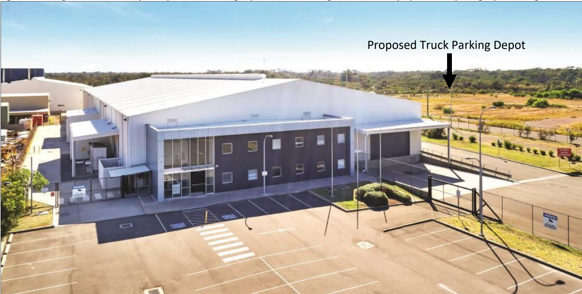
Figure 2.1. Tomago Resource Recovery Facility and Truck Parking Depot – front of Building 1 and location of proposed truck parking depot in background.
