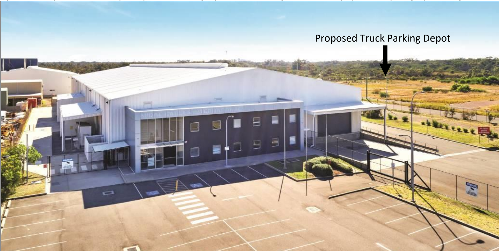
Figure 2.1. Tomago Resource Recovery Facility and Truck Parking Depot – front of Building 1 and location of proposed truck parking depot in background.
