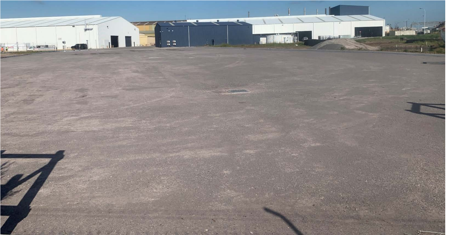
Photograph 2: View from the eastern end of the truck parking area
