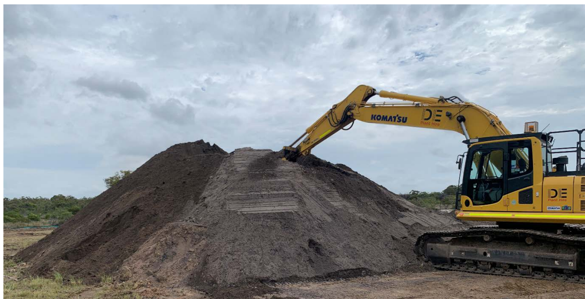
Photograph 3: Sampling Zinc stockpile SP1, 16 December 2021.
