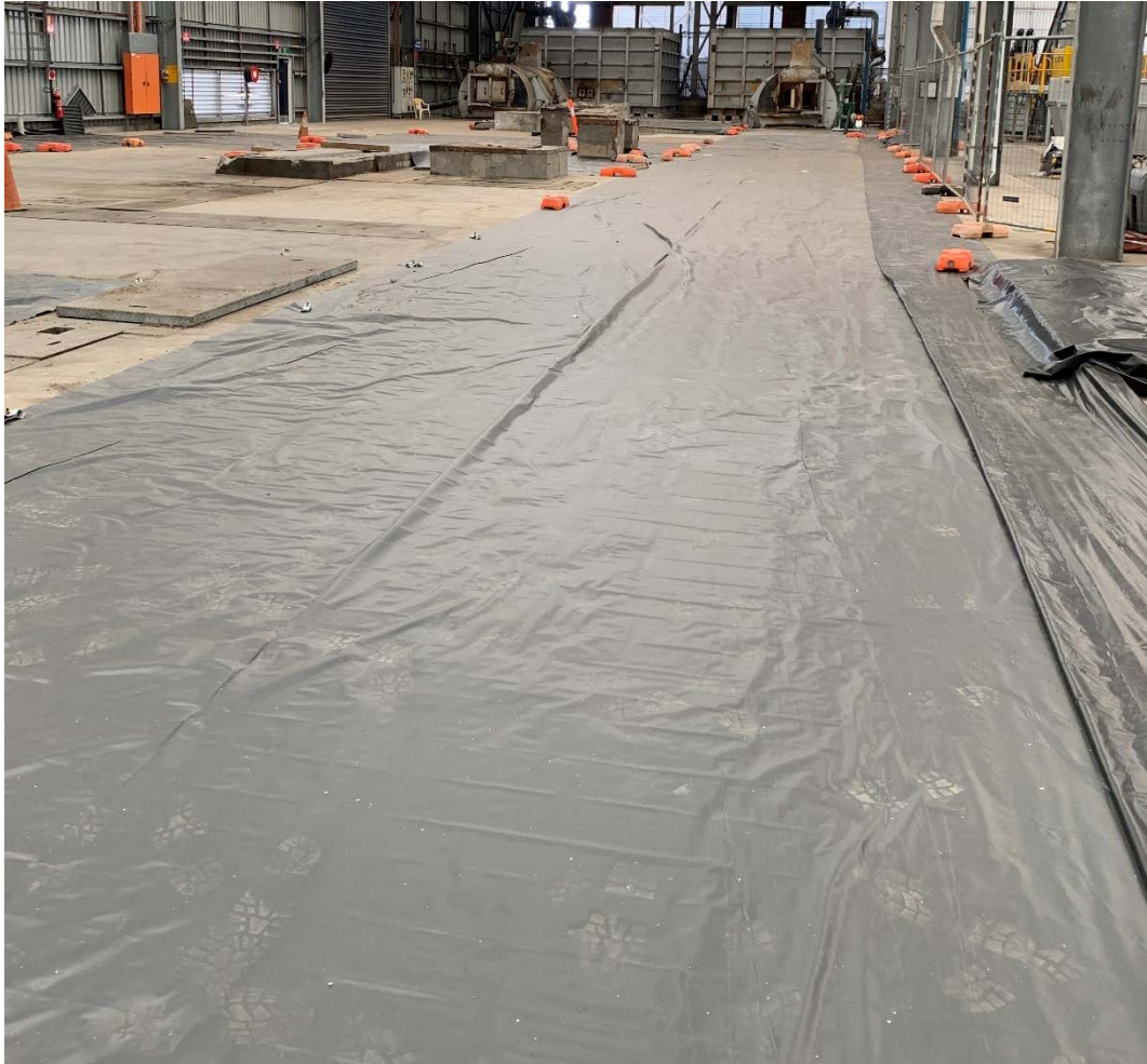
Photograph 3: Plastic covering Concrete Pit 2.
